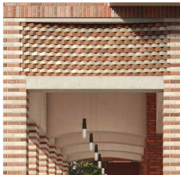
Detail of woven brickwork from proposed project
