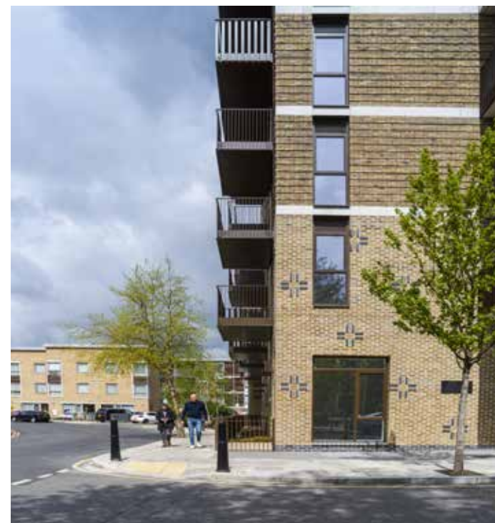
Above: Barchester Street by Metropolitan Workshop Illustrating effect of changing mortar colour using same brick
