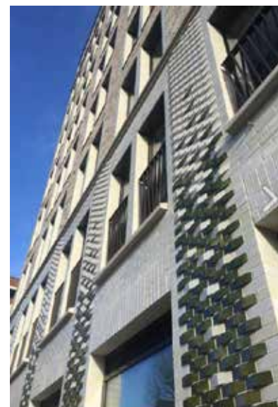
Weave brick pattern using saddle back bricks to plinth
